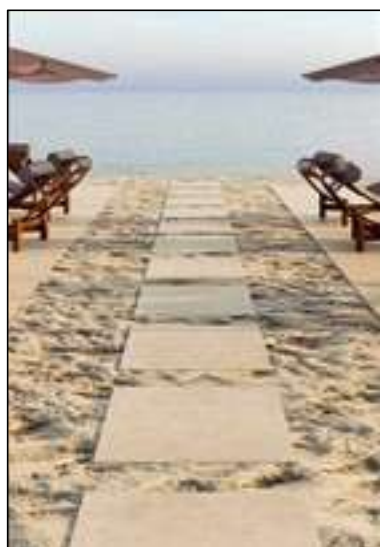
DRY INSTALLATION ONTO SAND pag. 68
